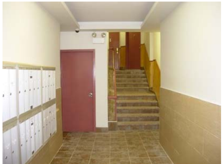
After renovation, the lobby of 60 Hester Street now sports new mailboxes, a new door, reinforced paint work on walls and railings, as well as a security system.
